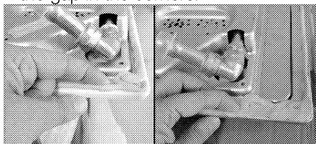
**i** Make sure that the skirting sections on the lower housing of the hob are filled with putty.
